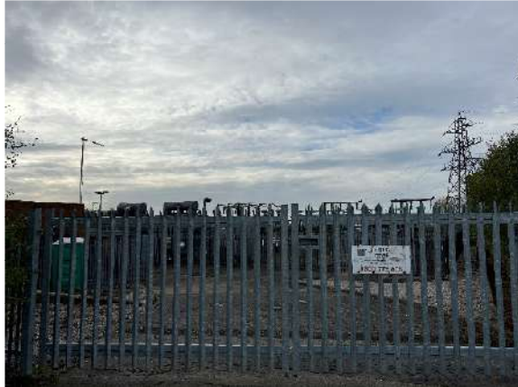
Plate 33 - Area 11 Substation adjacent east boundary
