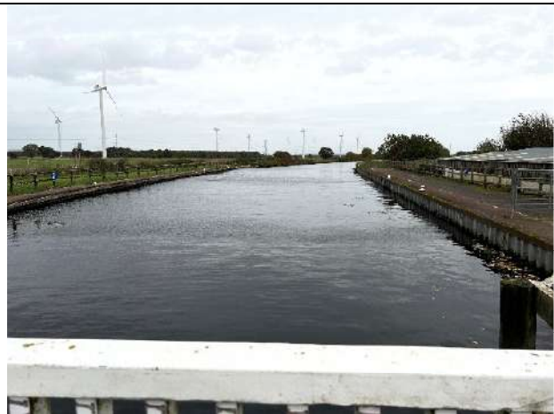
Plate 30 -Area 8 Mauds Bridge over Canal looking east
