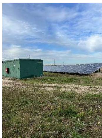
Plate 32 - Beyond Area 11 northeastern boundary Thorne Solar Farm
